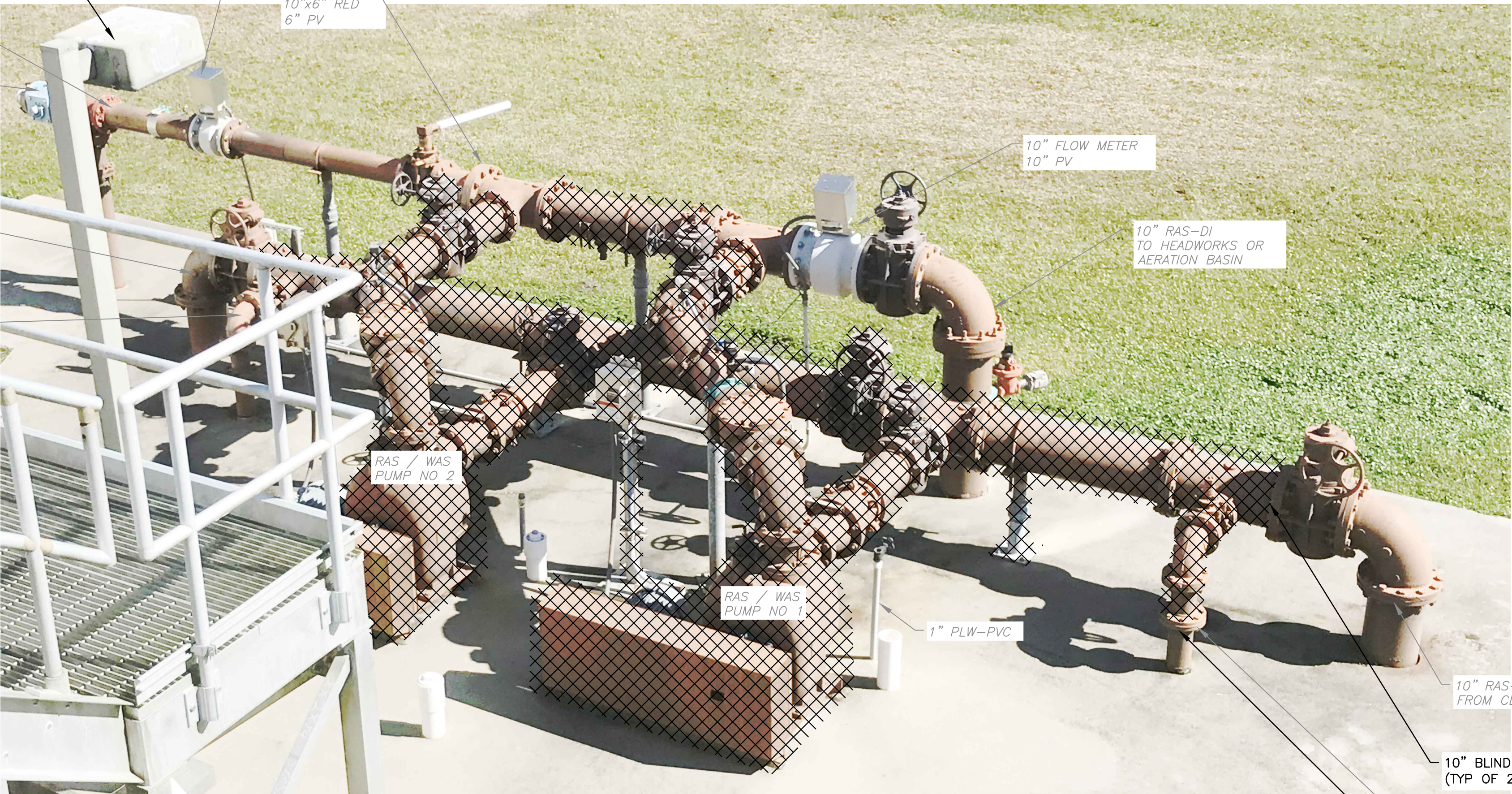
EXISTING RAS/WAS PUMP STATION DEMOLITION
